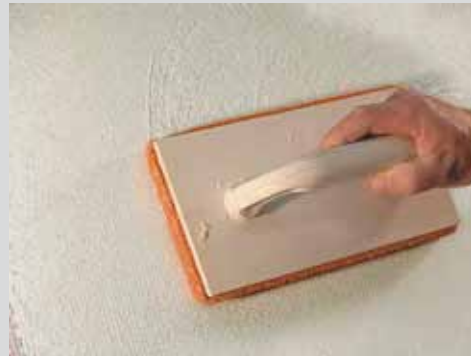
4 Rubbing in with coarse sponge float
