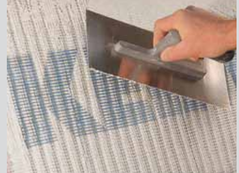
2 Optional placement of mesh
